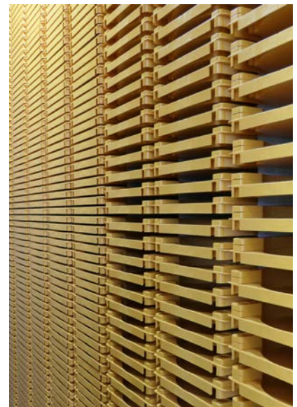
View into the tower
